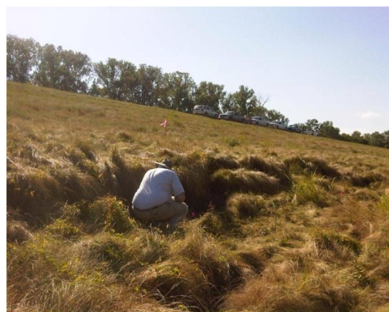
Figure 2. A typical levee slide. This one appeared in the spring of 2011
